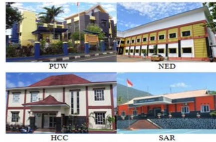
Fig. 4. Building Condition of the Study Object.
